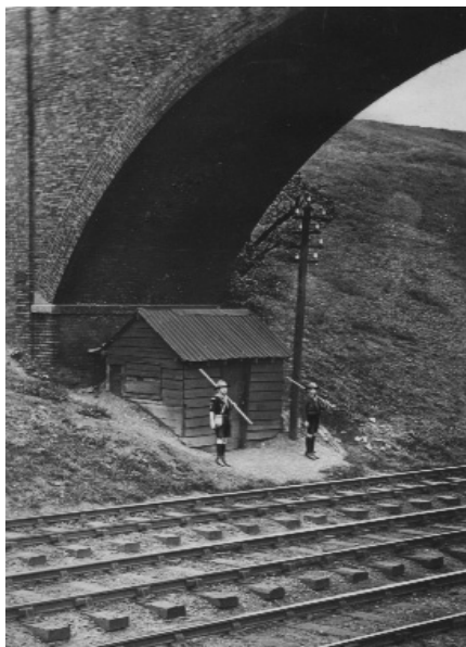
Guarding a Railway Bridge
