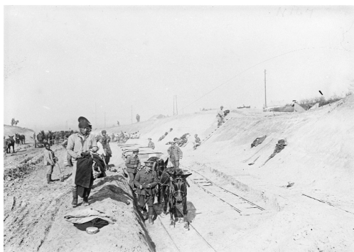
Canadian railway troops and Chinese labourers constructing a cutting at Lapugnoy, March 1918. IWM Q10733
