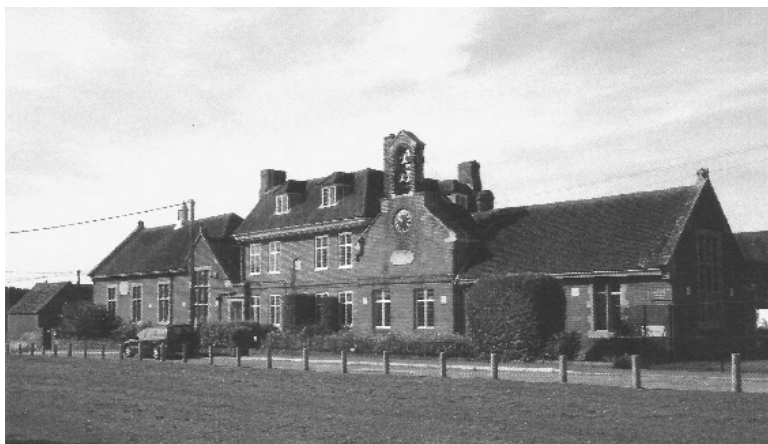
Piggatt's Charity School, Shinfield. The four-bay central section is the original building. It was extended in the nineteenth century. photo David Cliffe
